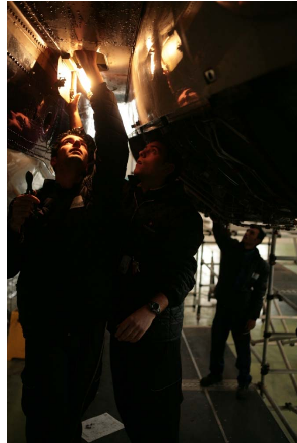
Electrical, Hydro-mechanical and Environmental systems
