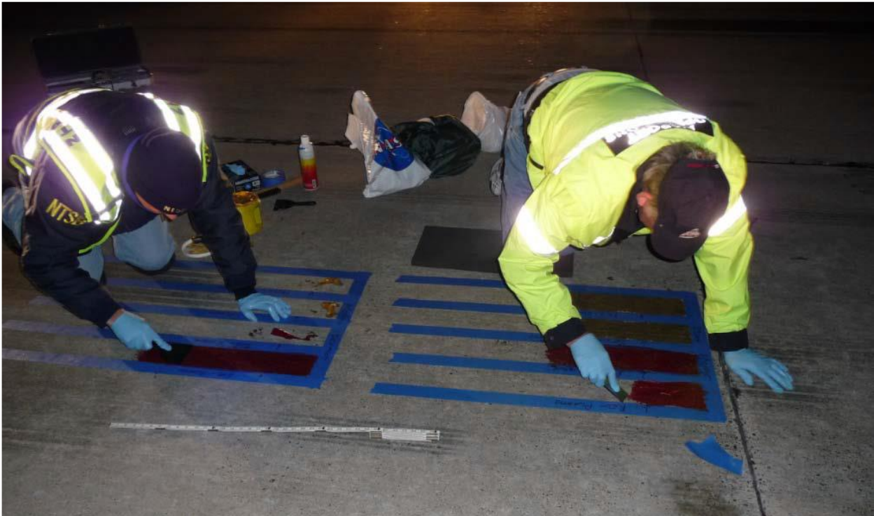
► Figure 4-5 Example of conducting grease test (Source: NTSB)
