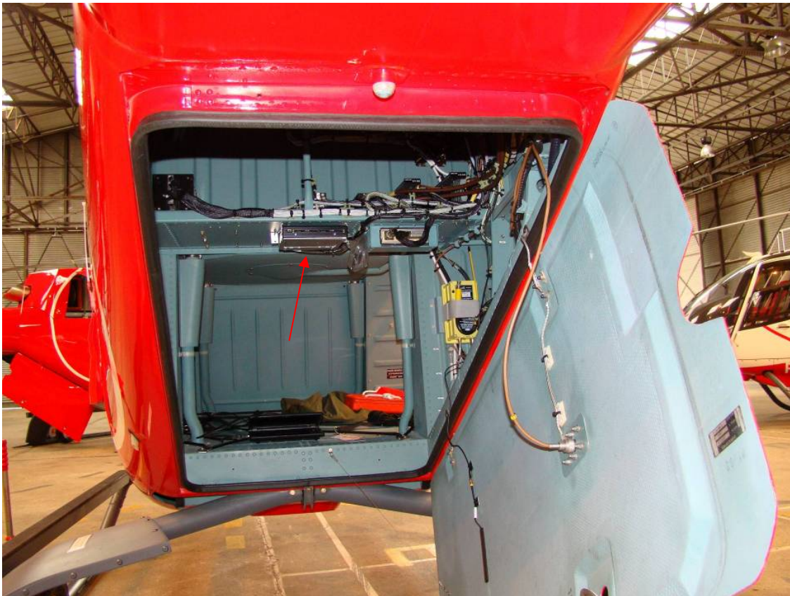
Picture 2 – installation on EC120
